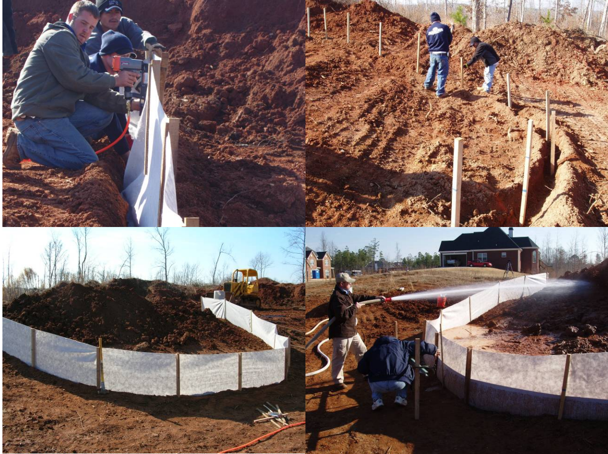
Figure 18 Installation of the BSRF for field testing.
