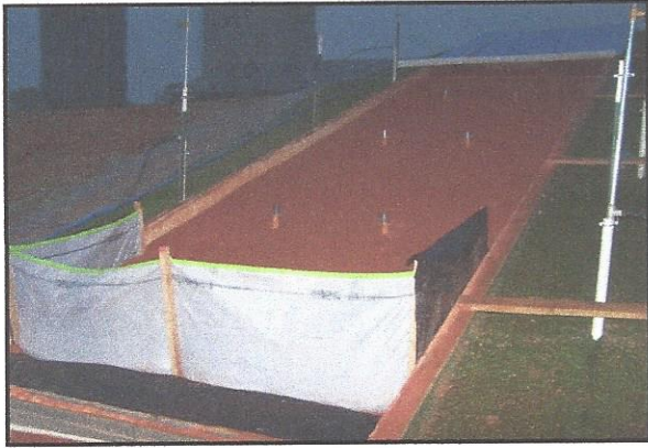
Test Slope Prepared and Fence Installed
