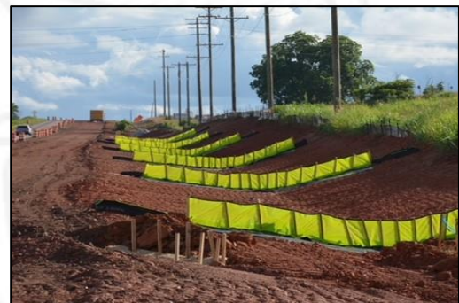
Natural floatables contribute to filtration on green mesh of velocity restrictor sheet
