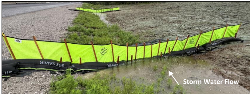
HVDC 24 for flat bottom, trapezoidal ditch
