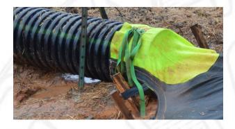
**Step 4.** The Slope Drain Bag has 8 loops for stakes. We only stake 7 of those loops. The bottom low side loop is left open for bag expansion.
