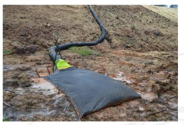
**Step 3.** Attach Slope Drain Bag to HDPE Pipe 12" or smaller using the straps provided.
