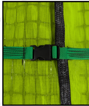
1" buckles secure pedestal wrap to inlet
