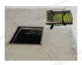
Step 4. Place 2x4, rebar or pole into handles.
