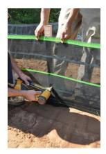
It is important for structural integrity to use the >350 lb. belts as attachment points to the wood posts.
