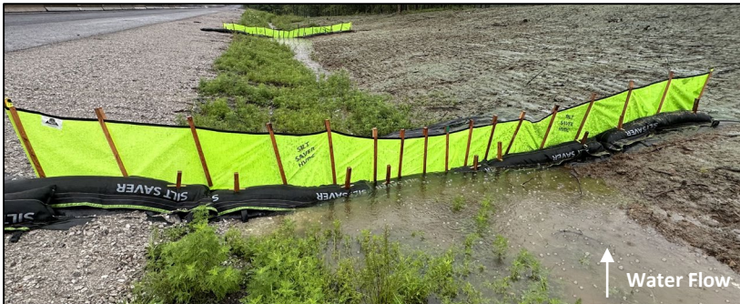
Front water seal with compression tubes and stakes
