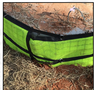
"D" rings secure pedestal wrap to inlet
