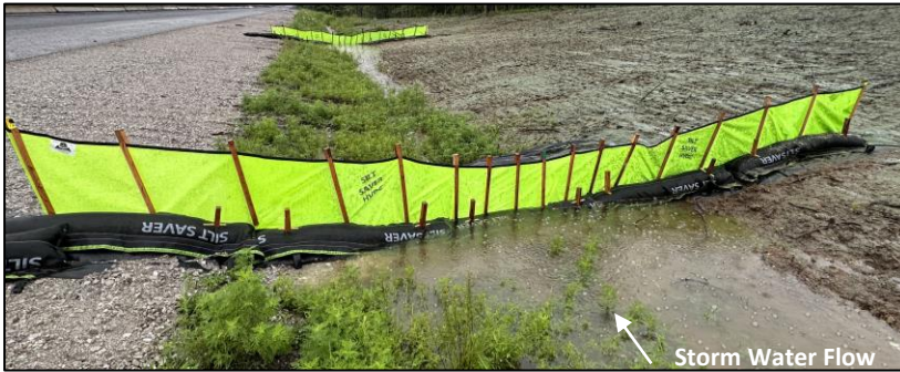
HVDC 24 for flat bottom, trapezoidal ditch
