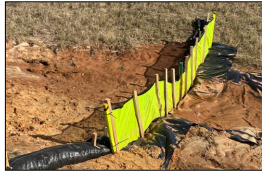
HVDC 14 for V shaped ditch
