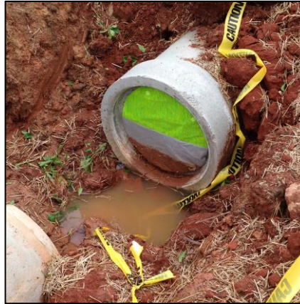
Friction fingers clip into HDPE, Concrete, or Metal Corrugated Pipe
