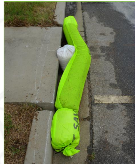
Single SS 300s for 5' inlet opening Use of center weir recommended
